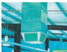
Straight Modular Supply system with high velocity discharge.
